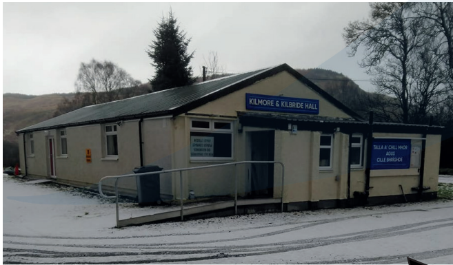
Before repair and extension works were carried out
